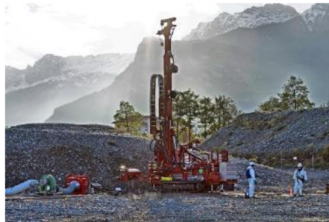
Complex sonic drill rig
