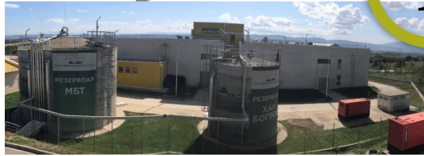
The WWTP of the Solid waste treatment plant of Sofia
